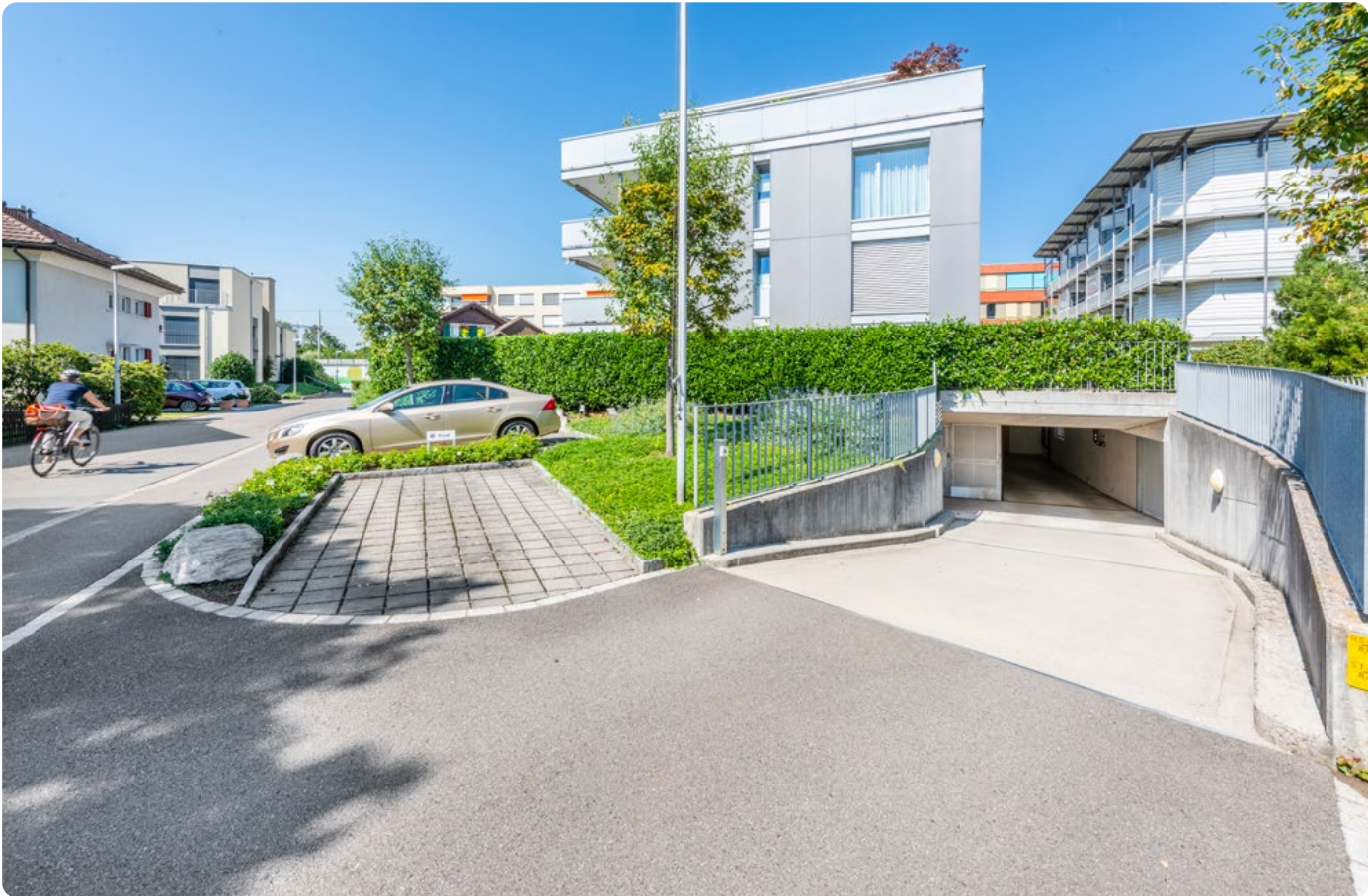
Underground garage entrance
