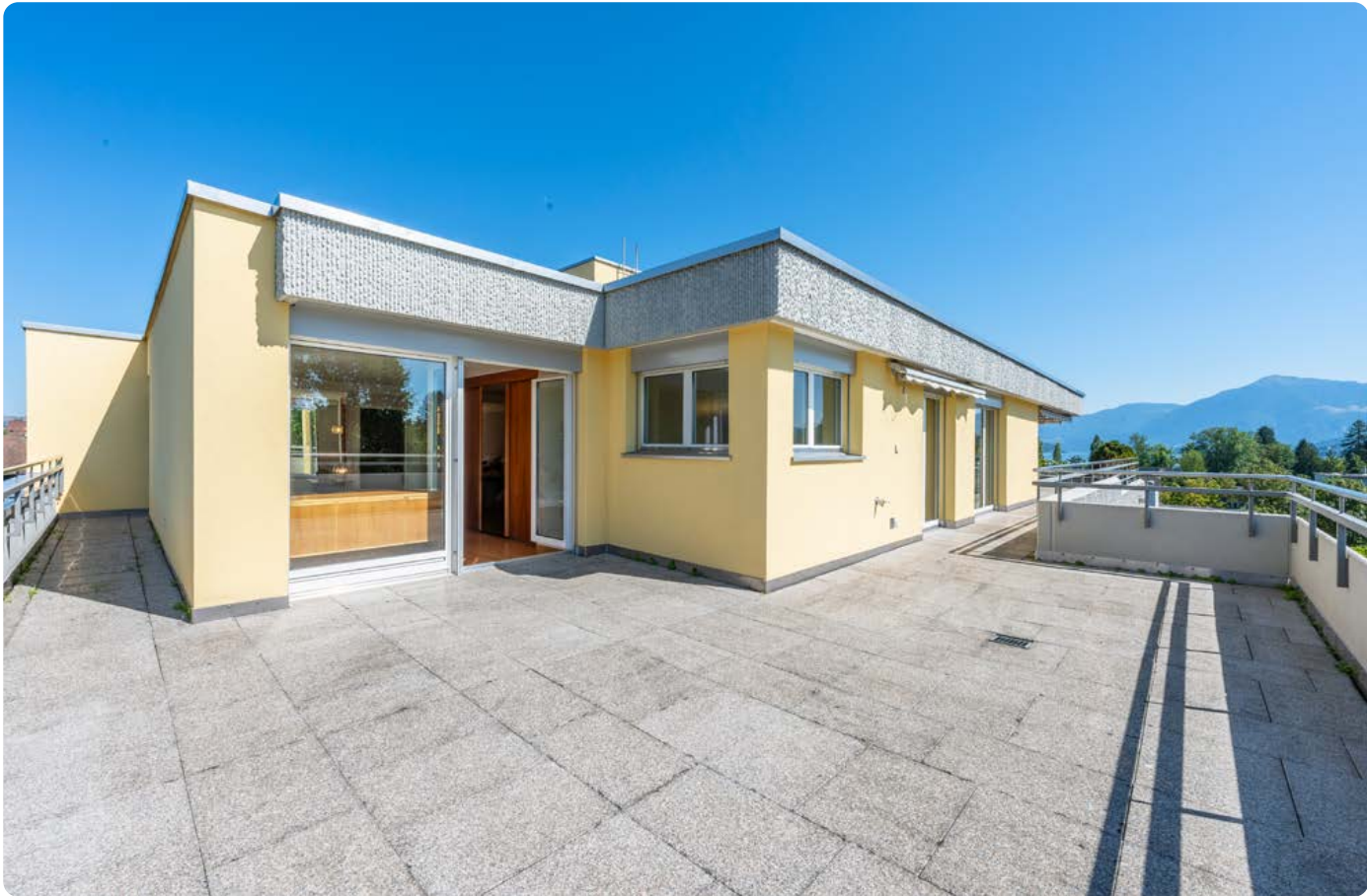
Terrace on the northwest-facing side
